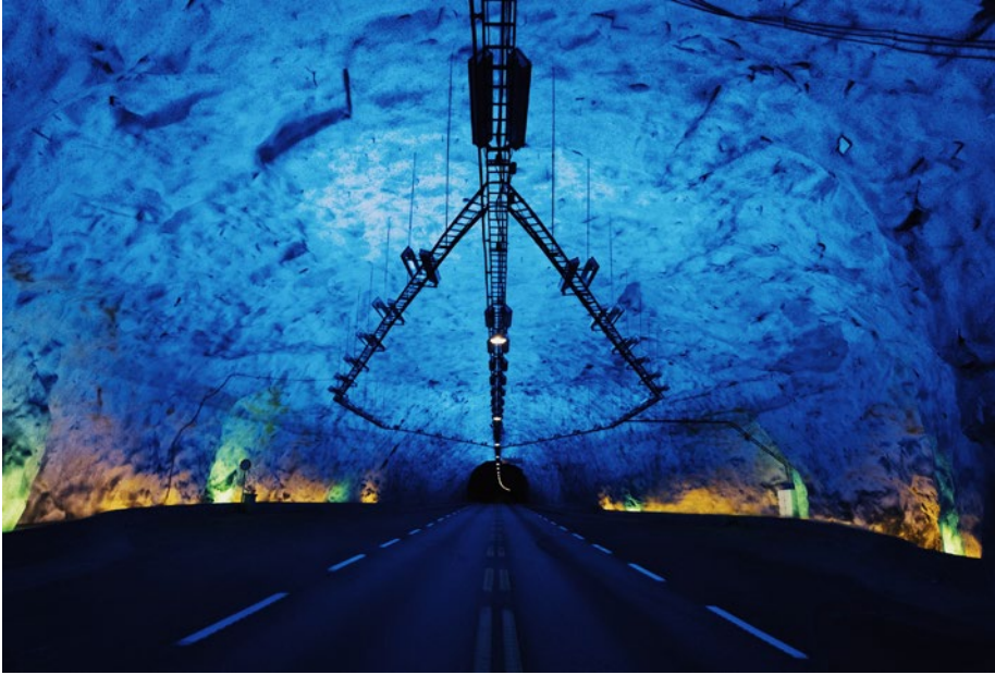
Figure 30-1. Lærdal tunnel's illuminated caves 3
